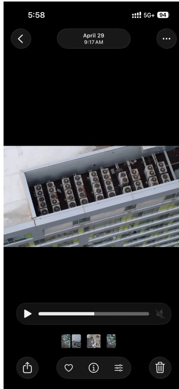
Drone photograph, April 29, 2026 9:17 AM EDT. Building rooftop mechanical well showing stacked per-unit outdoor condensing units. Visible rust streaks and water staining on multiple cabinets indicate deferred maintenance across the equipment fleet.
